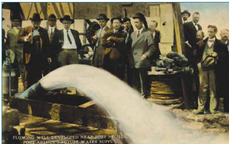
FIGURE 9. Flowing artesian well developed for the Port Arthur, Texas, water supply (circa 1910).
