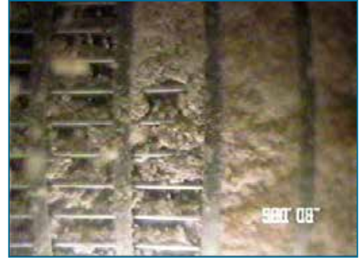
FIGURE 39. Scale formation on a well screen. (Source: Gary Hix)
