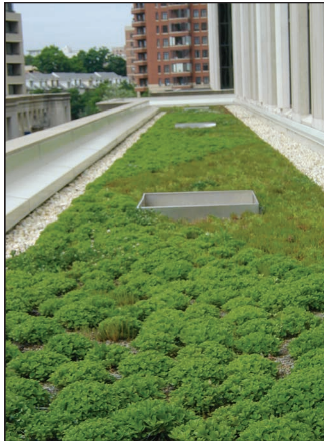
Figure 41. This green roof constructed on top of a building acts as a bioretention system. (Photo courtesy of Joan Kelsch, Arlington County Government.)
