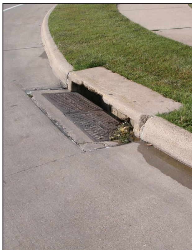
Figure 42. Regular cleaning and maintenance of streets can help minimize pollutants that enter storm drains in urban areas. (Photo courtesy of Nikki Dictson, Texas AgriLife Extension Service.)
