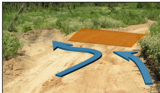
Figure 50. Waterbars and wing ditches help to safely drain road surface runoff water to prevent erosion. (Photo courtesy of the Texas Forest Service.)
