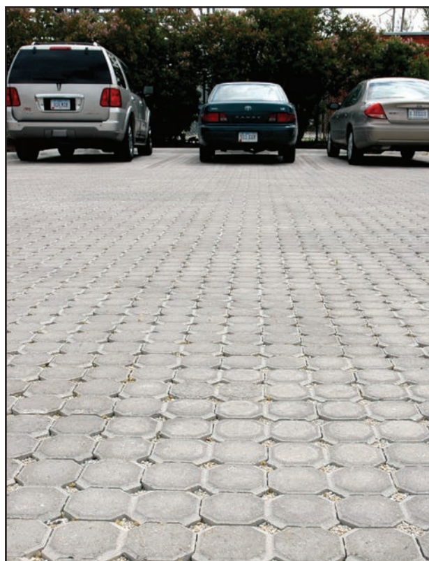
Figure 38. A porous pavement system in a shopping mall parking lot. (Photo courtesy of USDA Natural Resources Conservation Service.)
