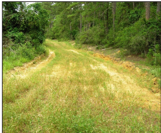
Figure 47. Revegetation stabilizes disturbed soil and prevents erosion. (Photo courtesy of the Texas Forest Service.)
