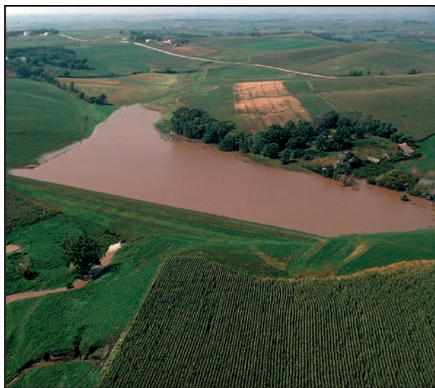
Figure 34. Water and sediment control basins hold runoff water to prevent flooding and sedimentation. (Photo courtesy of USDA Natural Resources Conservation Service.)
