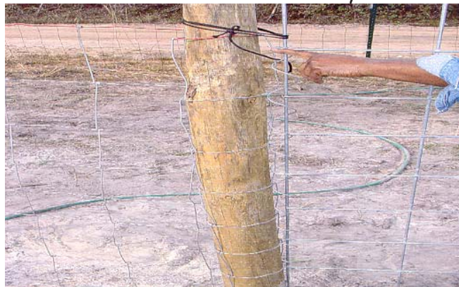
Fig. 20 Use nylon rope to secure the panel to the post.
