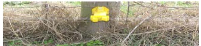
Fig. 13 A insulator used to support the electric wire.
